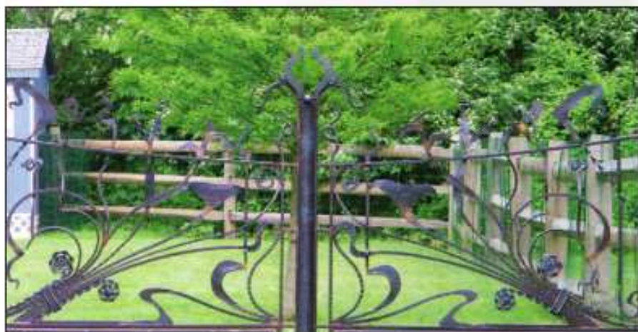
Framework and finish. The bottom panel is hammered copper sandwiched between round bar that was forged to an un-uniform 1/2 round to give a wing or web feel. The whole gate is mounted on an I-Beam that runs column to column. Finish is natural. Approx. labor time: 120 hrs.
